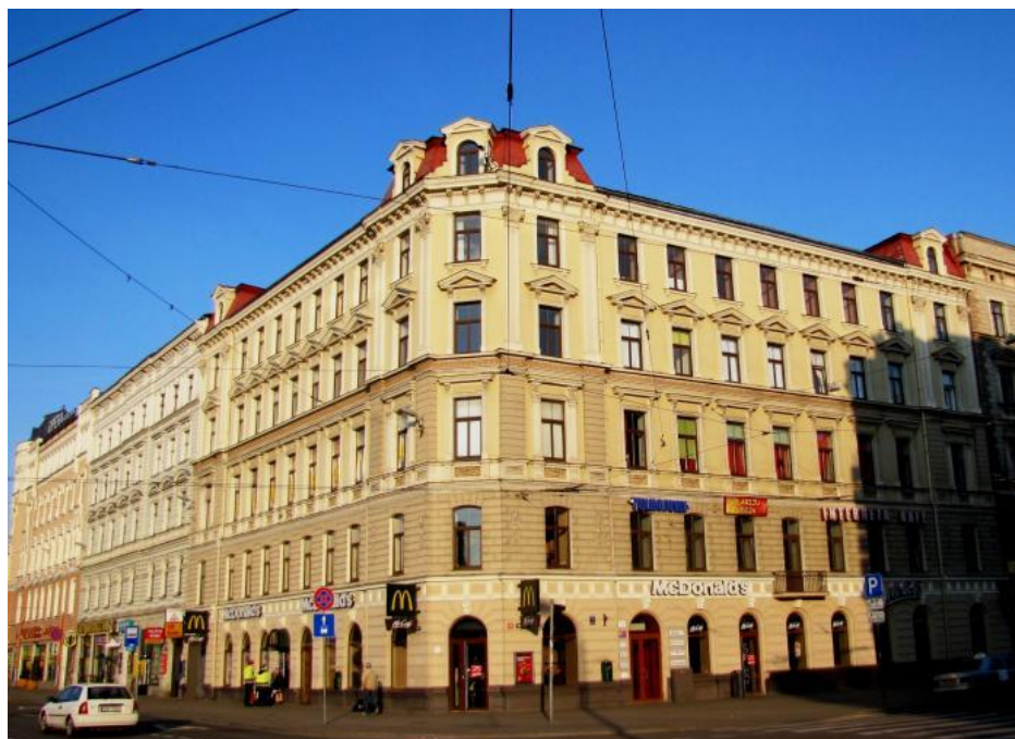
Commercial & office building – Merkela Street, Riga, Latvia
